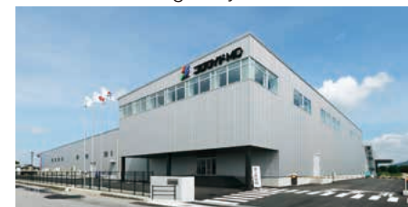
COLOWIDE MD Co., Ltd. Nagahama Central Kitchen
