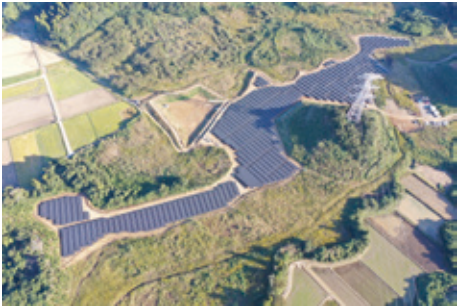
Solar power plant in Chiba Prefecture
