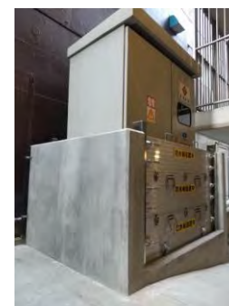
Installation of water stop
