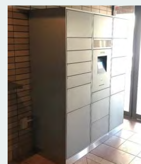
Installation of additional parcel boxes
