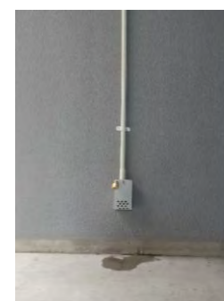
Installation of flood sensors
