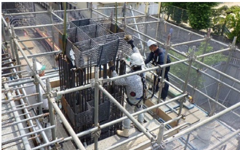
Arrangement of high-strength shear reinforcement (civil engineering / elevated rail bridge)
