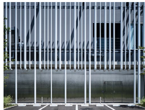
Louvers Used as Rainwater Gutters
