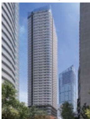
Atago District Category 1 Urban Redevelopment Project F District
