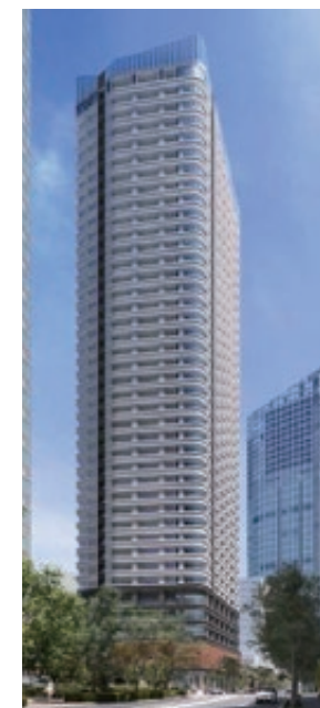
Atago District Category 1 Urban Redevelopment Project F District
