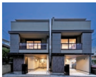
Shibuya Sasazuka Station w5 Project
