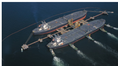
Tugboats help a very large crude carrier (VLCC) to berth at the Keiyo Sea Berth
