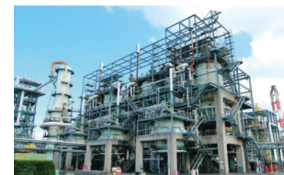
Vacuum residue thermal cracking unit (Eureka Thermal Cracking Unit) of Fuji Oil
