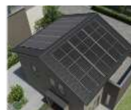
Residential solar power system installation
