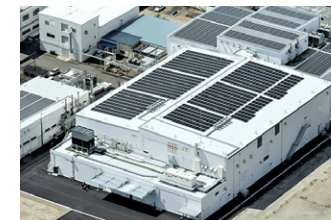
Expanded clean plant (Konan Plant)
